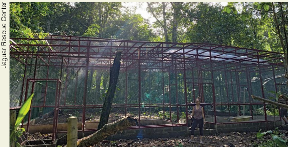
Newly built enclosure
